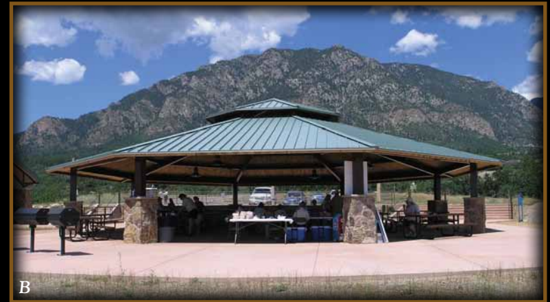
B Cheyenne Mountain, Colorado Springs, CO: 58'-6" Savannah model 12" o.c. standing seam steel roof, 4:12 pitch, in Hemlock Green color. 2" x 6" cedar T & G sub-roof & cedar fascia.
