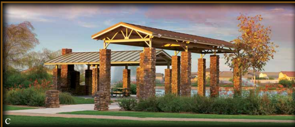
C Rancho El Dorado, Maricopa, AZ: Custom 13'-8" x 46' & 20' x 32' Orlando models are centerpieces located at the entrance of a new upscale housing community. Custom masonry & faux stone surrounds underlie an I-beam frame and a Marine Green standing seam steel roof with tubular steel fascia.
