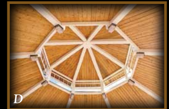
D T & G subroof and no exposed conduit to interior lighting.
