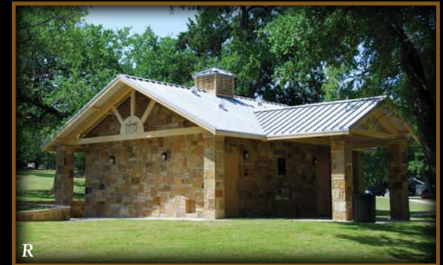
R Finch Park, McKinney, TX: 32'-6" x 38'-6" T-shaped Campion model w/ Metallic Silver standing seam roof w/ Beige powder coat.
