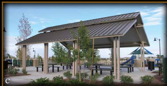
Walton Park, Verrado, AZ: 26' x 34' Cheyenne model with 12" o.c. standing seam steel roof in "Weathered Copper" color. Features double tube steel columns with rafter extensions.
