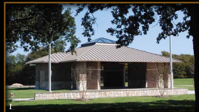
Rolling Oaks Memorial Center, Coppell, TX: 47'-10" x 61'-5" Custom Mesa pavilion w/ cedar T&G sub-roof under standing seam steel roof.
