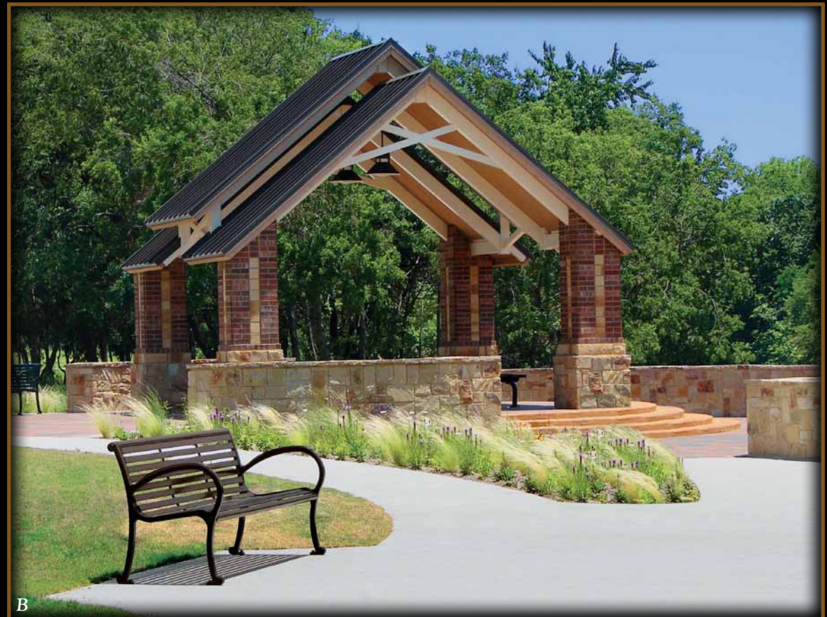
B Markwood Park, Irving, TX: 20' x 20' Aspen model with 12" o.c. Weathered Copper color standing seam steel roof with a 2" x 6" T & G sub-roof. Stone and brick by others.
