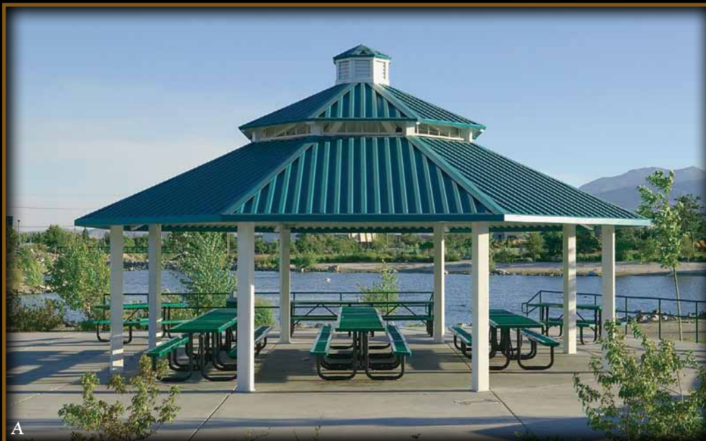
A Paradise Park, Reno, NV: This 28' model two-tier structure features a New England style cupola, with HR-36 roof, colored Jade Green.
