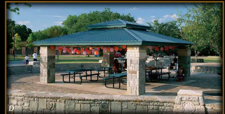
Hurwitz Park, Irving, TX: A beautiful 24' x 24' model w/ Tahoe Blue HR-36 steel roof, over 2" x 6" tongue & groove subroof. Masonry and stone work by Owner.
