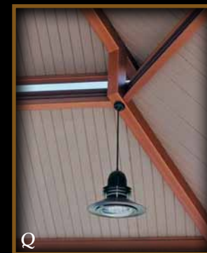
Dallas light detail, shown with 2" x 6" tongue & groove subroof
