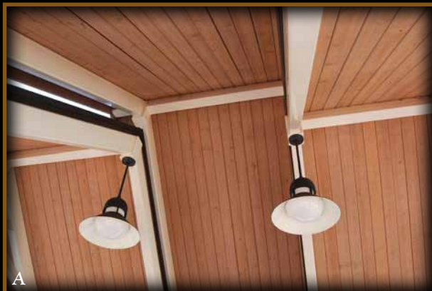
A Ceiling Detail: Select 2" x 6" T & G sub-roof w/ lights & hidden wire runs.
