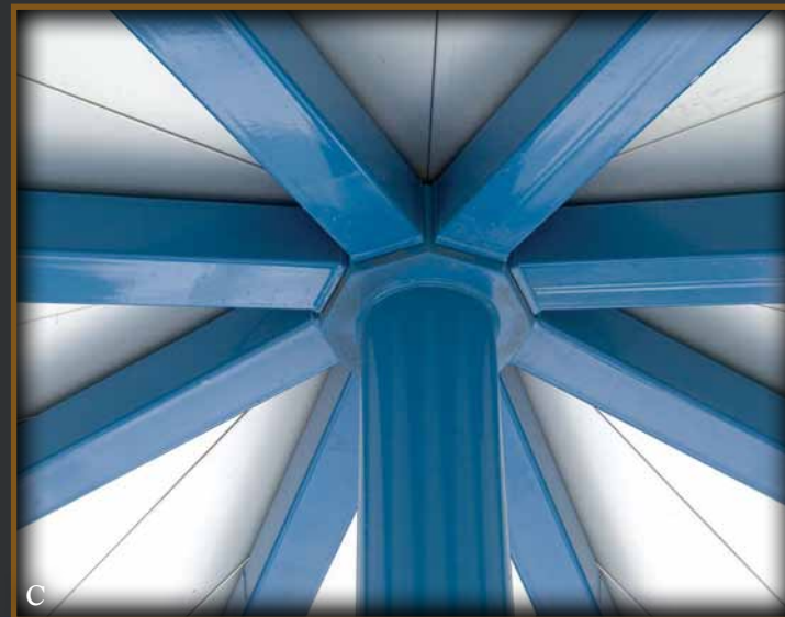
Meadow Woods Park, Orlando, FL: Detail of Hawaii model w/ 10" diameter post, hidden beam connections and smooth white standing seam underroof.
