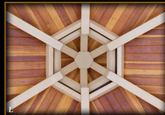
Custom cedar 2" x 6" T&G detail on Dallas model with cupola.
