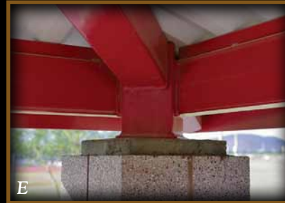
Denver column connection detail
