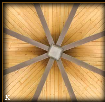
Standard tongue & groove and lighting detail.
