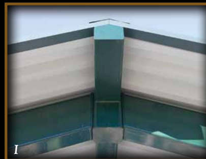
Standard Orlando model roof peak compression ring, rafters and extension beam detail
